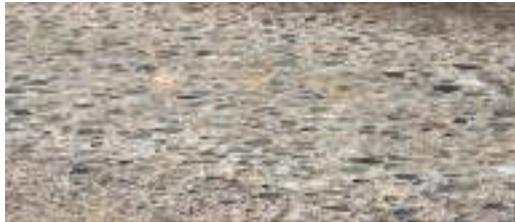
**Gambar 12.7:** Closed polished surface (Pemeliharaan Jalan, 2017)
